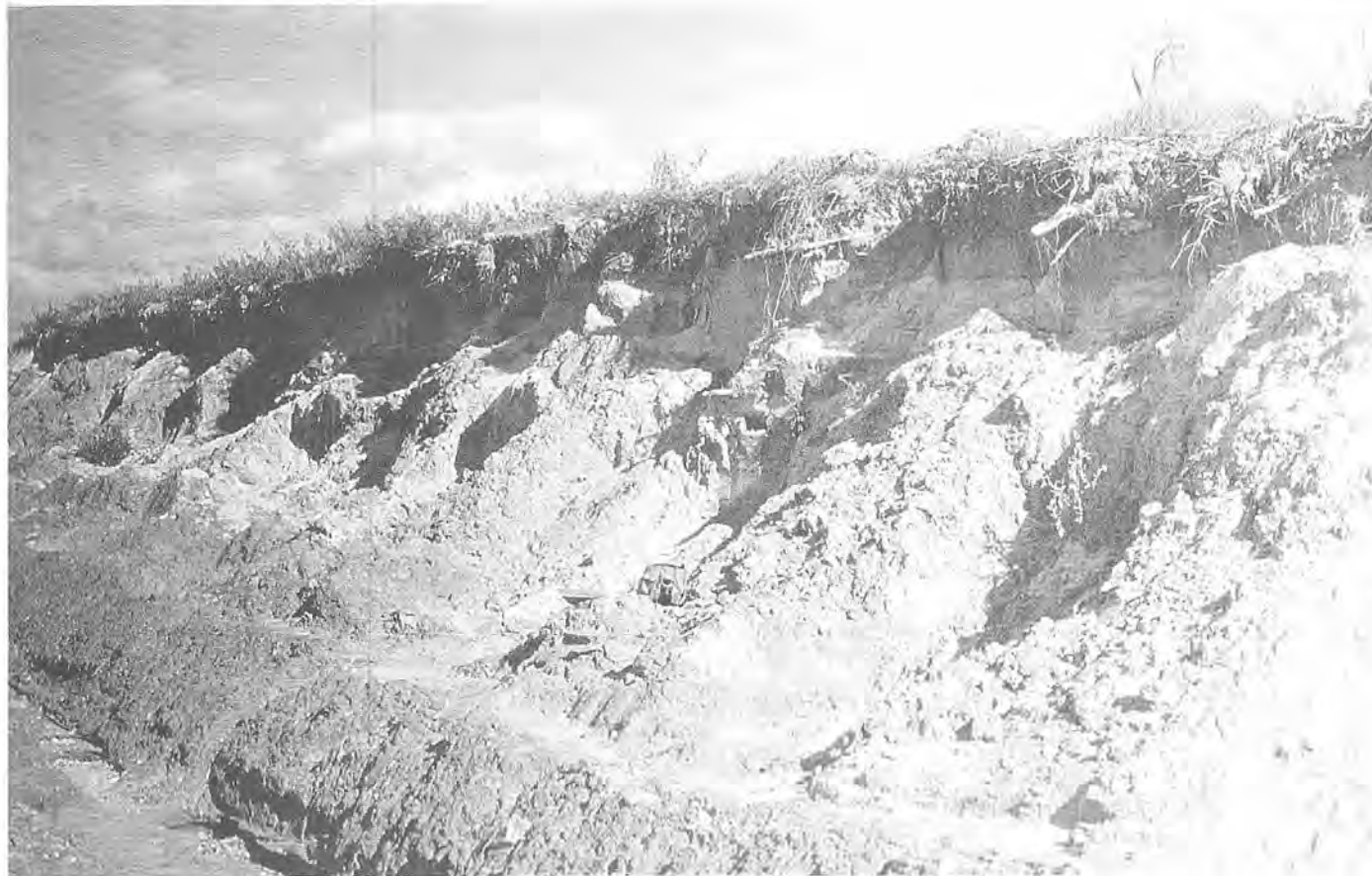
Plate 1. Road cut along Monkton Ridge Road near Winona Lake.
